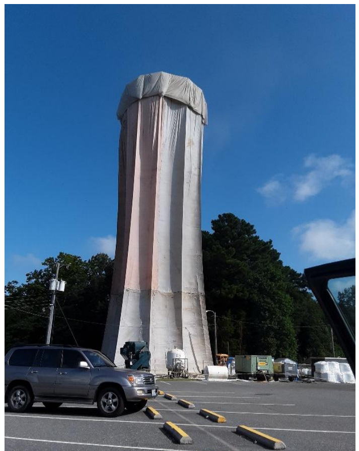
Kilmarnock Water Tower During Sandblasting
